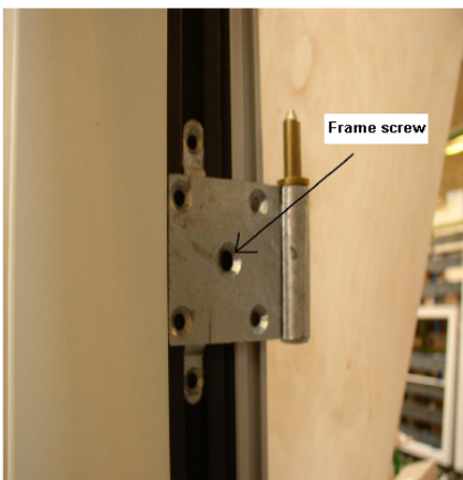
Figure 9. Mounting the doors
